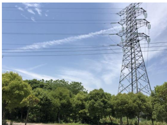
拟建雨泾 1391 汇龙支线拟建终端塔处
